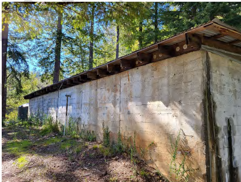
Photo 6: Buckeye Tank walls and general tank condition
