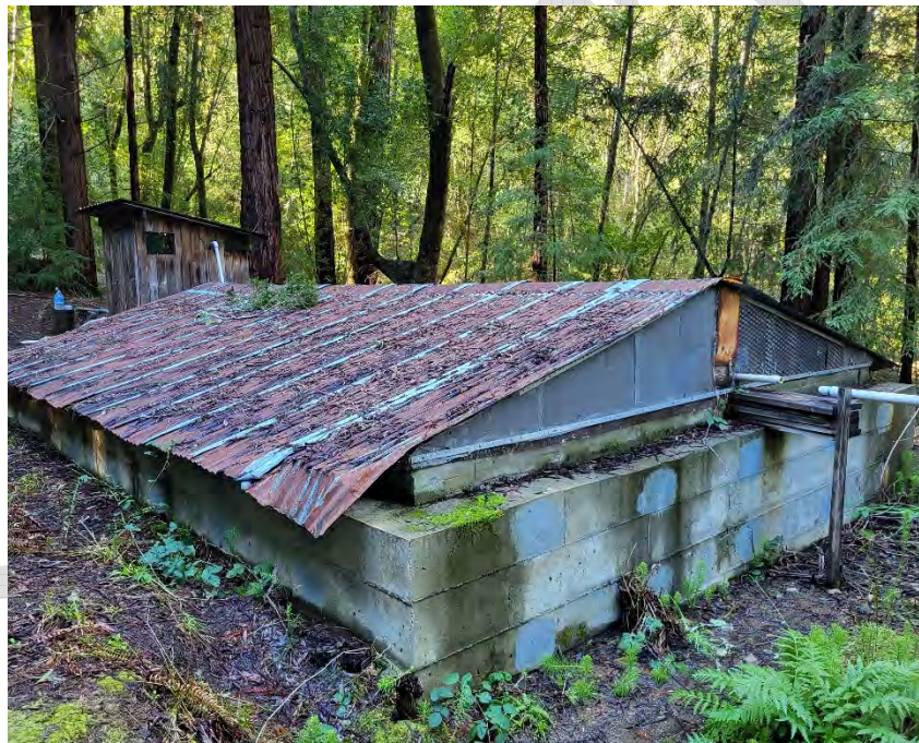
Photo 7: Hotel Tank general condition
