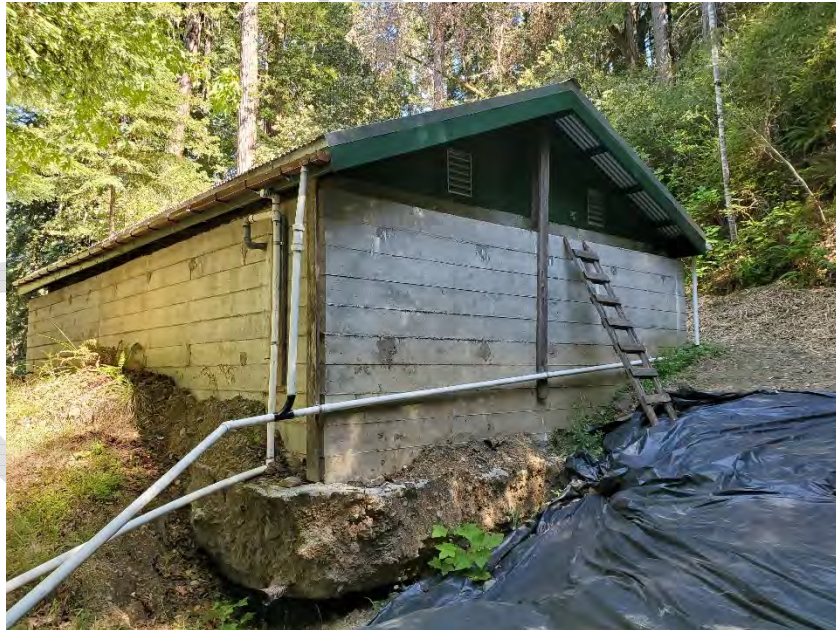
Photo 9: Void under the Luther Tank foundation
