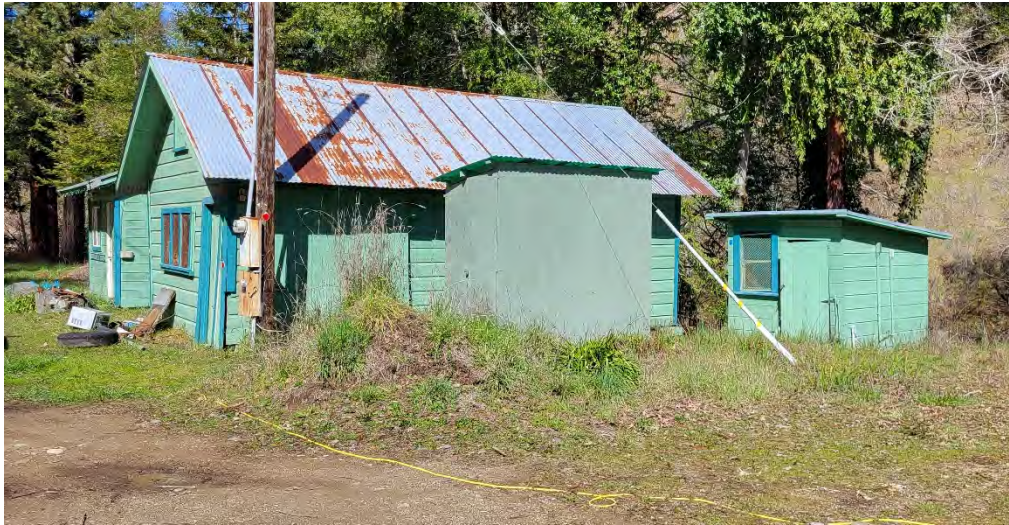
Photo 12: Existing Well Site storage shed (with gabled metal roof)
