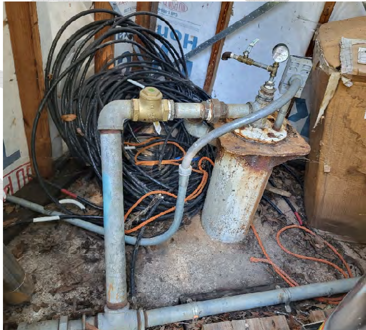
Photo 11: Hotel wellhead and surface seal condition
