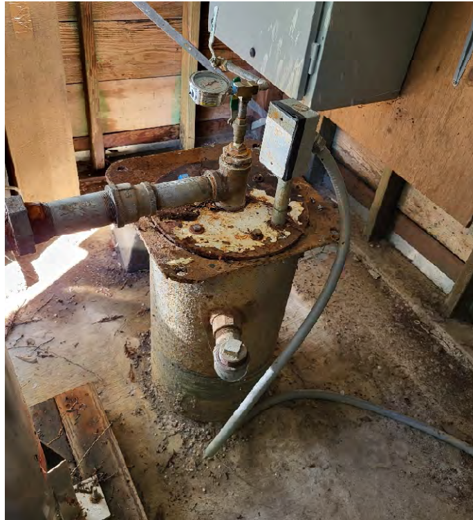
Photo 11: Hotel wellhead and surface seal condition
